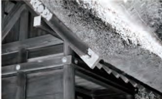
Thatch is still used in Japanese traditional architecture for pitch roofs.
